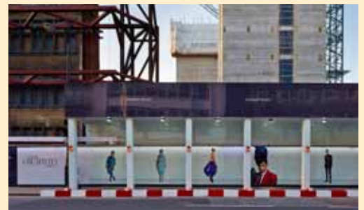
The new pedestrian gantry on the Mortimer Street elevation.
