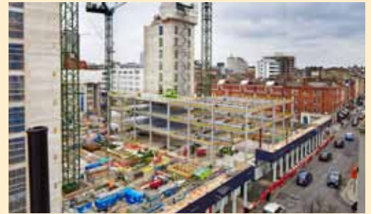
Office blocks to the Mortimer Street elevation under construction.
