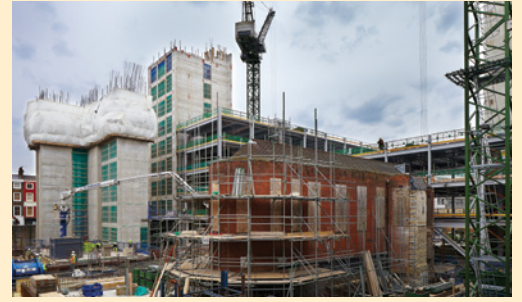
Scaffolding 'bird cage' under construction around the Chapel.
