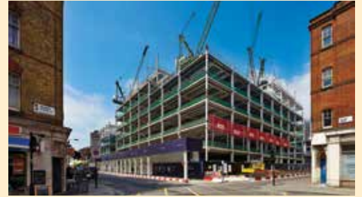
View from Mortimer Street and Cleveland Street junction.
