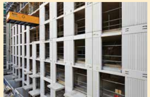
Inside the site, the cladding panels progressing on Block 5.
