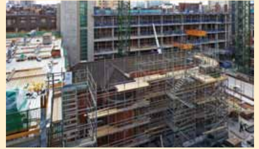
Scaffolding 'bird cage' construction progressing around the Chapel.
