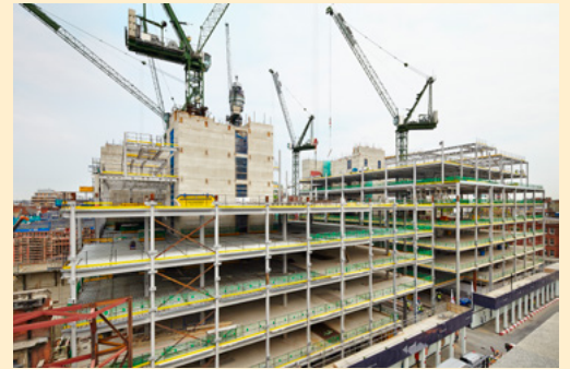
Aerial view from Mortimer Street.
