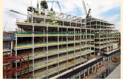
Aerial view from Mortimer Street.
