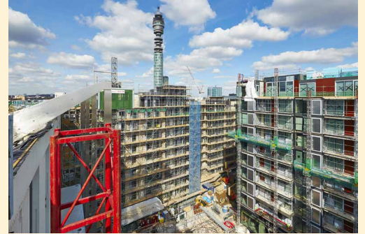
View of the courtyard looking towards the BT tower.
