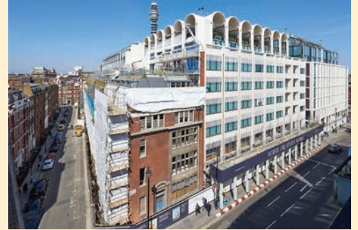
View of Nassau St & Mortimer St.
