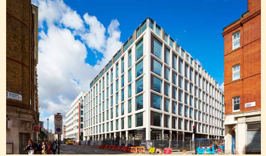
Office Block 1 – cladding completes
