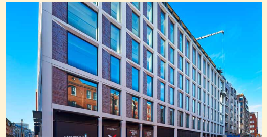
Office Block 1, Cleveland St elevation
