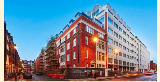
Office Blocks 1 & 2 from corner of Mortimer St & Nassau St
